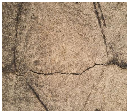
Minor cracking to the driveway
