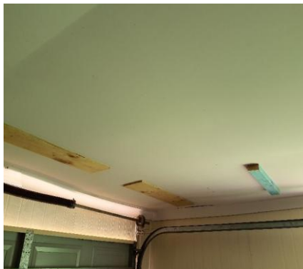
Timber has been attached to the garage ceiling
