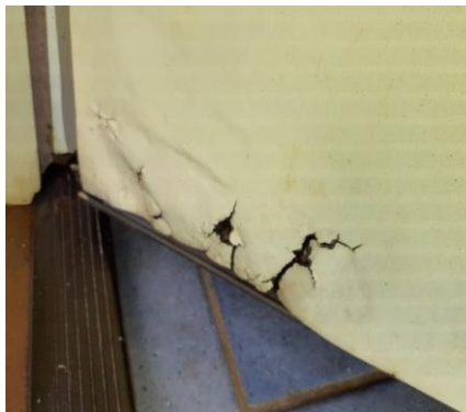
Water damage to the laundry external door
