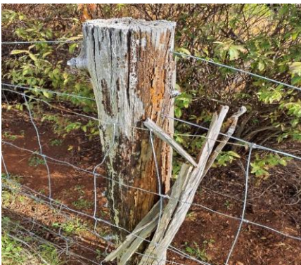
Wood decay to fence timbers
