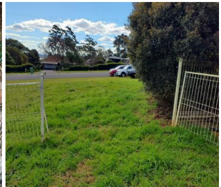
Fence gates are not attached
