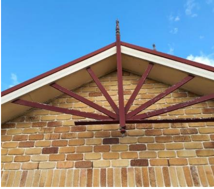
Wood decay to timber mouldings in the gable
