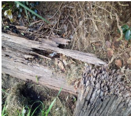
Wood decay and termite damage to retaining wall timbers
