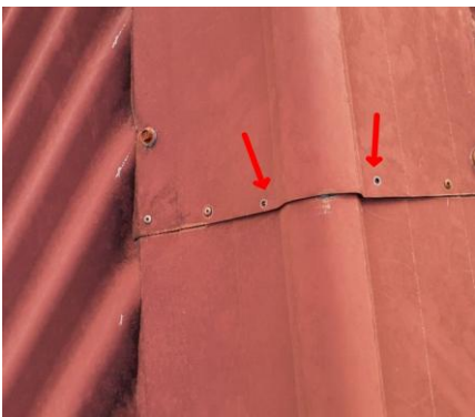
Pop rivets missing from join of ridge capping
