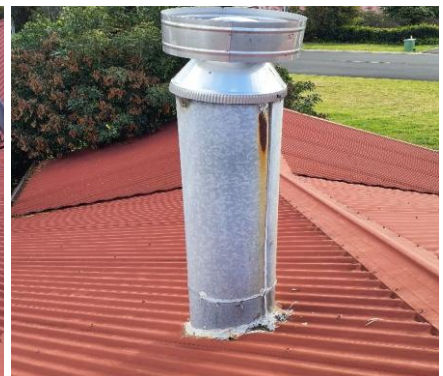
Minor rust and there is no boot around the flue
