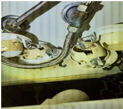
Rust to flexible hoses under the kitchen sink
