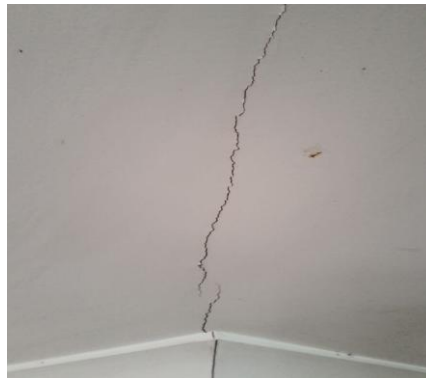
Cracking to the lounge room ceiling
