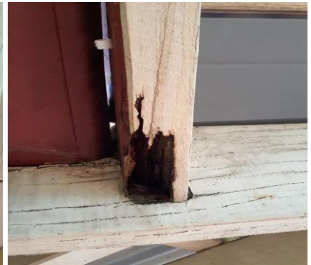
Wood decay to patio structure framework
