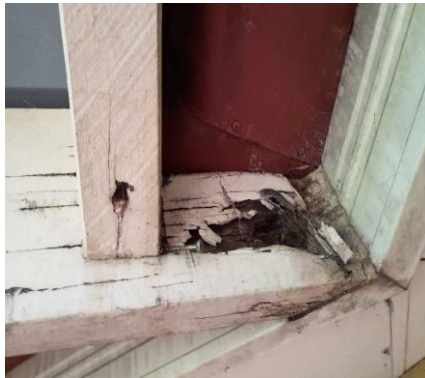
Wood decay to patio structure framework
