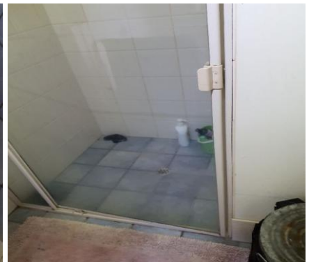
Shower screen door is not closing fully
