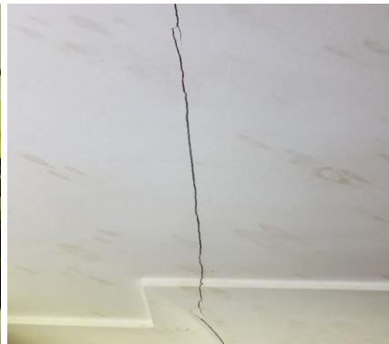
Cracking to the join of the dining / kitchen ceiling
