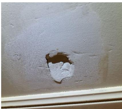
Damage to hallway wall lining
