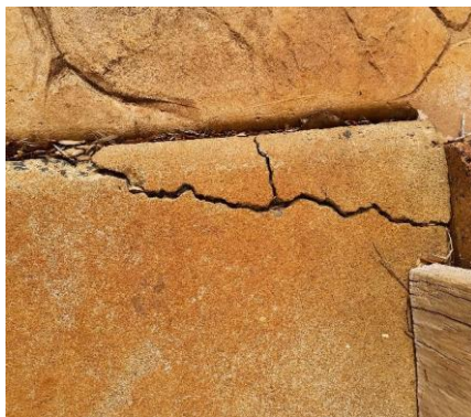
Cracking to the garage floor
