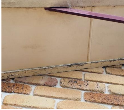
Weathering to the timber mouldings on eaves
