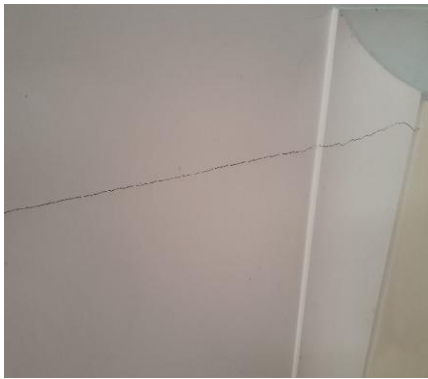
Cracking to the entry ceiling
