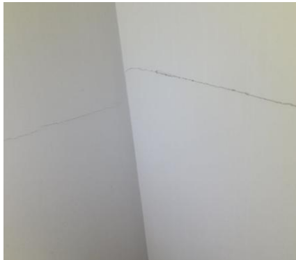
Minor cracking to the ensuite wall sheeting
