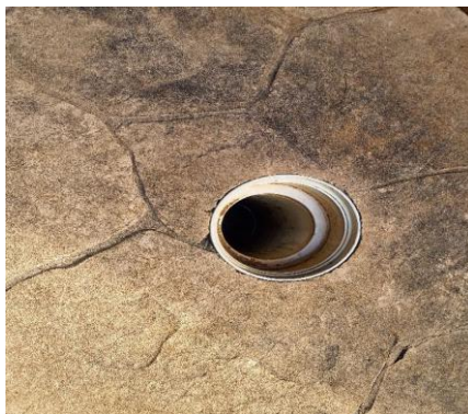
Grate is missing from drain
