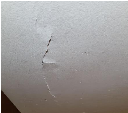
Damage to section of the lounge room wall lining
