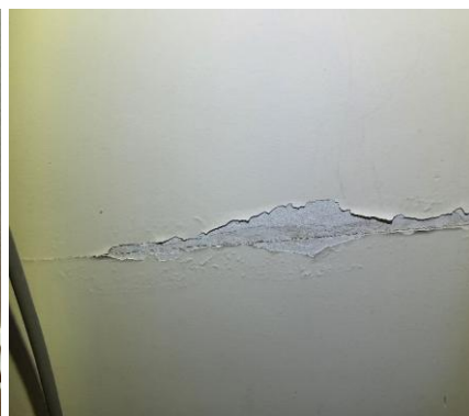
Cracking to join of the laundry wall sheeting and paint flaking
