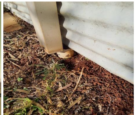
Shed downpipe is not connected
