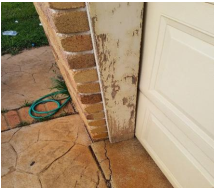
Weathering to the garage door frames
