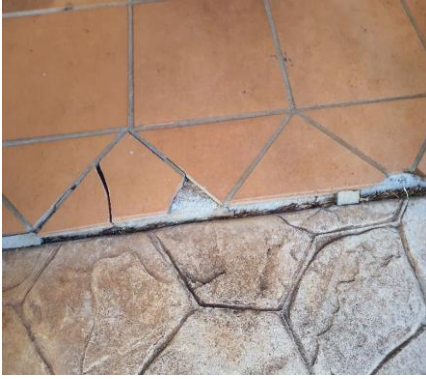
Damage floor tiles on the front porch
