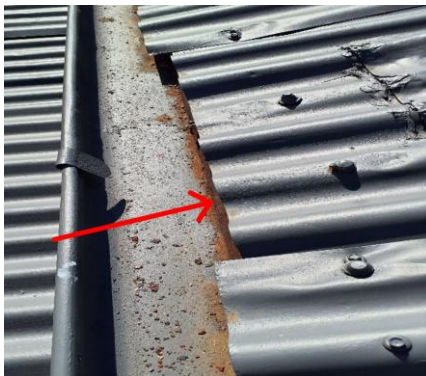
Roofing iron is short
