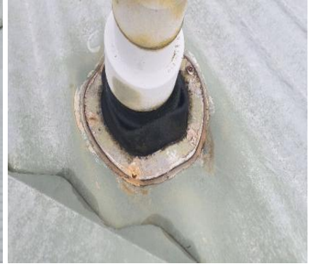
Sealant shows signs of deterioration around vent pipe boot
