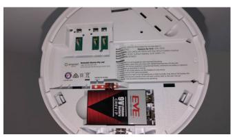
10: Emerald Alarms Cable Interconnect 240V Photoelectric Level 4 Top Of Stairs Apr 2033 Smoke alarm compliant: Smoke alarm upgrades a Clipsal 240V Ionisation smoke alarm.
