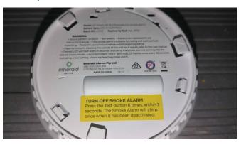
5: Emerald Alarms Wireless Interconnect Lithium-Ion Photoelectric Smoke alarm compliant: Smoke alarm was added to achieve compliance.
