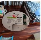
All smoke alarms located within the property as detailed above have been cleaned and tested as per manufacturers instructions and been installed in accordance with Australian Standard AS 3786 (2014) Smoke Alarms, Building Code of Australia, Volume 2 Part 3.7.2 of the National Construction code series (BCA) and AS/NZS 3000:2018 Electrical installations.
