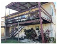
Severe wood decay is present to the structure. Repairs or replacement of some timbers will be required. The area is considered to be structurally unsound and the area should not be used until it is repaired and/or replaced.
