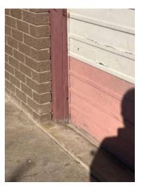
Some gutters and/or downpipes appear to discharge rainwater directly adjacent to the foundations of the structure. These should be connected to a stormwater dispersal system.
