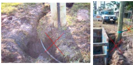
Above: Poles with become unstable if undermined
