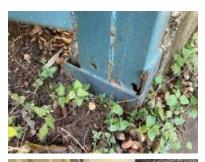
Cracked concrete stumps noted. The reinforcement steel to stumps is rusting and causing stumps to crack. This is considered a serviceability defect. Recommend a suitable experienced restumping contractor to further investigate and give probable cost of
