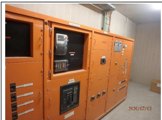
Main Switchboard (Lower Ground)
