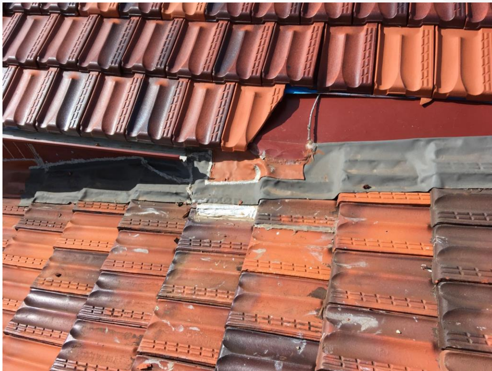
Poor flashings at junction Lot 6 to Lot 7
