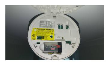
5: Clipsal Cable Interconnect 240V Photoelectric Smoke alarm compliant.
