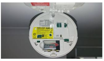
2: Clipsal Cable Interconnect 240V Photoelectric Smoke alarm compliant.
