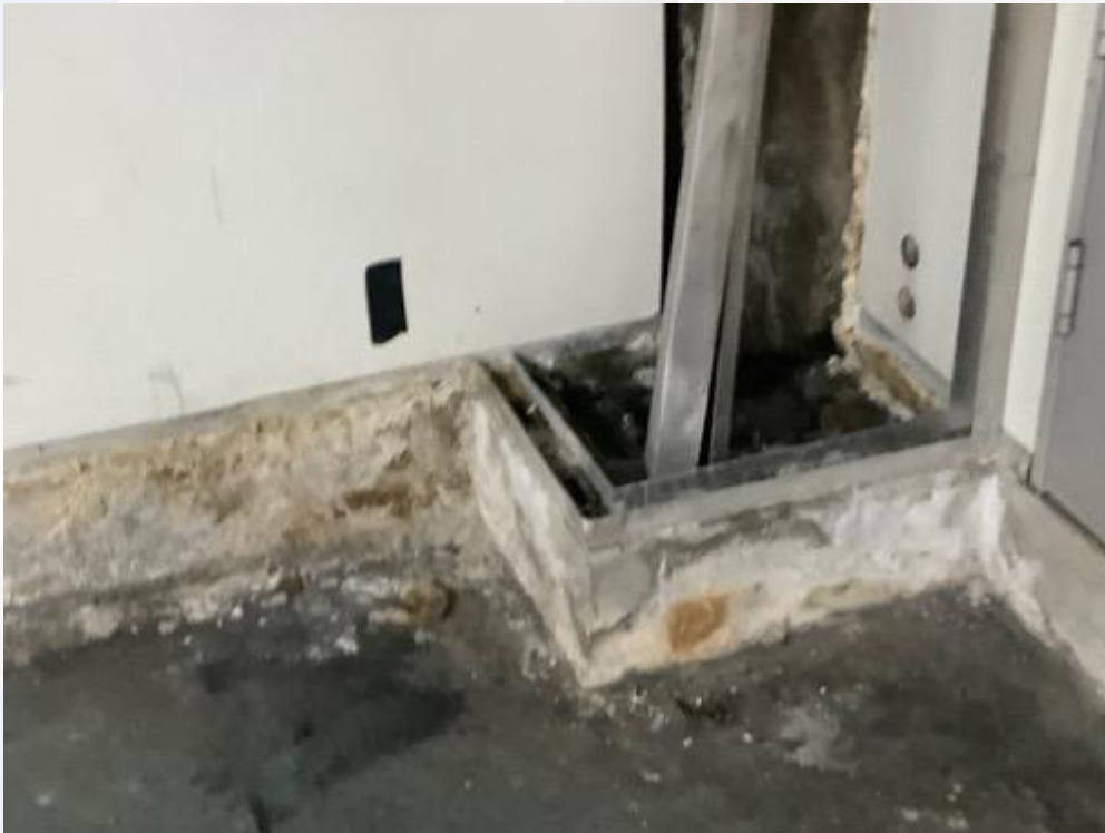
61. Water leaking through fan room wall and wet on the floor
