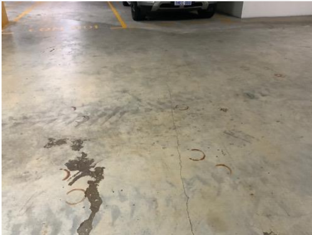
48. Cracking driveway west side opposite COMM G02
