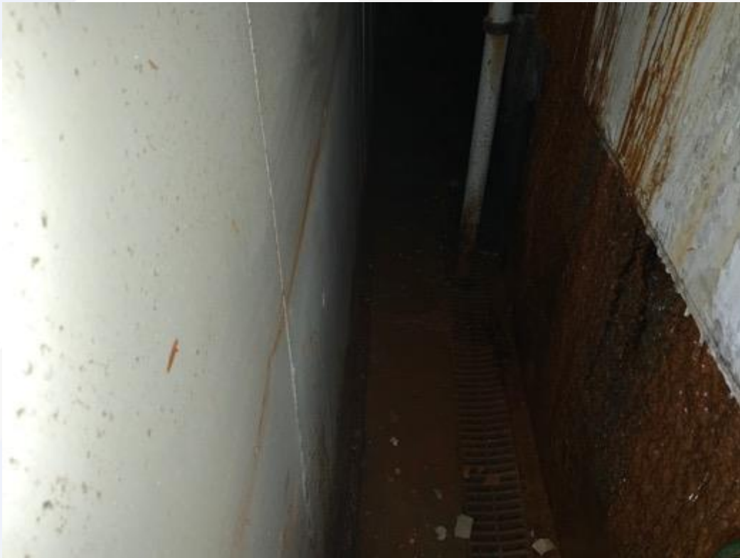
125. Salt build up to skirting to splay corner south east rear of car bay 502
