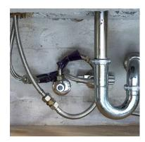
These flexi hoses have a limited lifespan, they wear out, or the nozzles that fit them to your incoming water connection can burst off, leaving you with your mains water supply running directly into your apartment.
