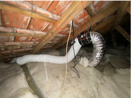
Bathroom extraction system ducting Ducting leads to exterior soffit. View High Resolution Image Here
