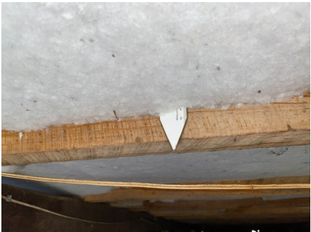
Sub floor Insulation Insulation measurement is 100mm. View High Resolution Image Here
