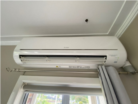
Heater Heat pump, Mitsubishi Current heater meets or exceeds the heating requirement. View High Resolution Image Here
