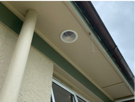
Kitchen extraction system external vent Confirmed by smoke test. View High Resolution Image Here
