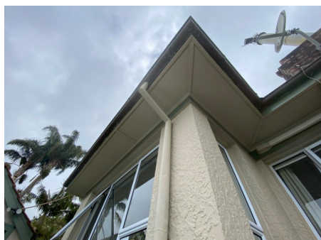
Right side of property - down pipe Down pipe is in good condition/ or near new condition and affixed securely to building. View High Resolution Image Here
