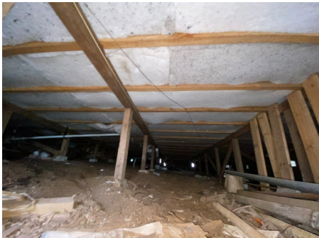
Sub floor Insulation Insulation is evenly distributed throughout sub floor. View High Resolution Image Here
