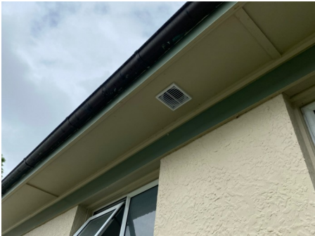
Bathroom extraction system external vent Confirmed by smoke test. View High Resolution Image Here
