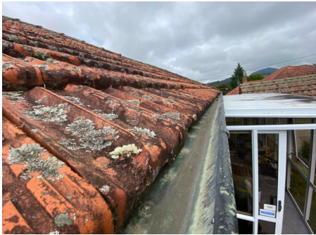
Rear of property - spouting Spouting is clear of debris. View High Resolution Image Here
