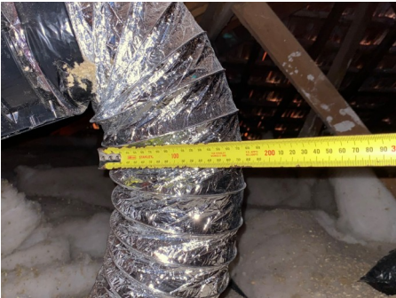
Bathroom extraction system ducting Ducting measurement is 120mm. View High Resolution Image Here
