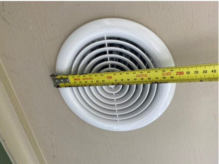
Kitchen extraction system external vent Vent measurement is 150mm. View High Resolution Image Here
