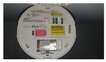
4: Legrand Cable Interconnect 240V Photoelectric Smoke alarm compliant.
