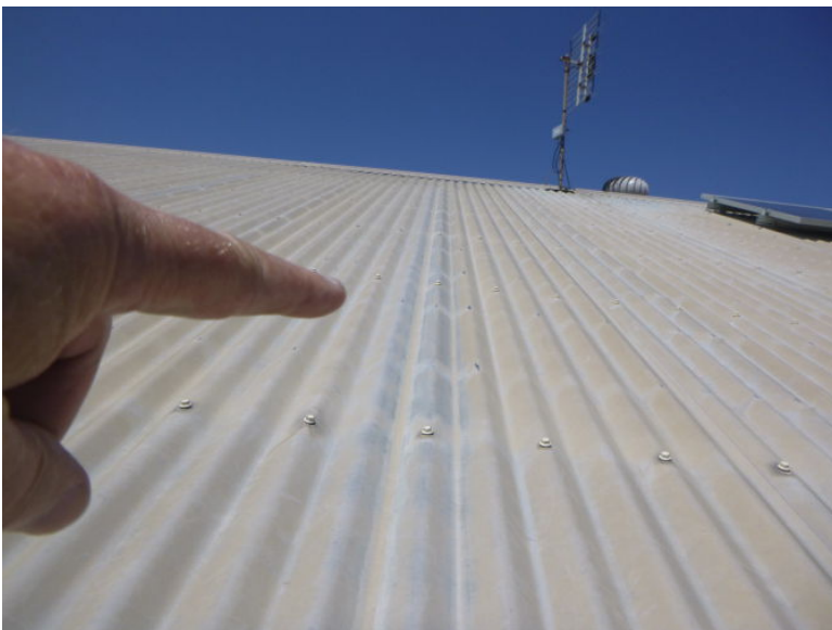
Image comments: UV degradation of the paint covering.
