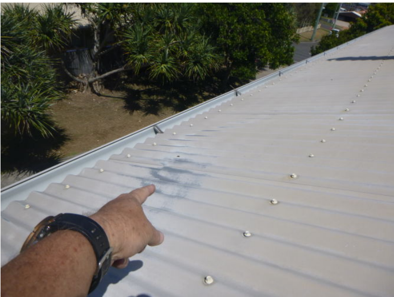
Image comments: UV degradation of the paint covering.
