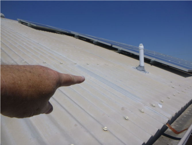
Image comments: UV degradation of the paint covering.
