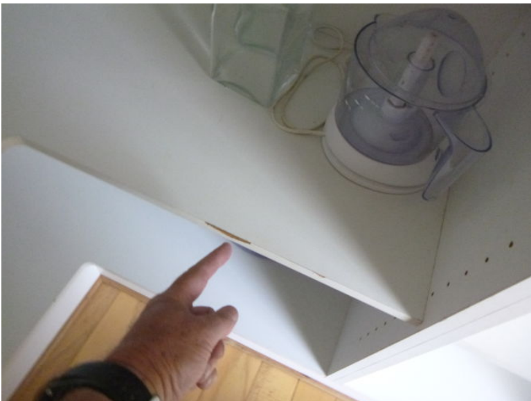
Image comments: Pantry shelf edge damaged.
