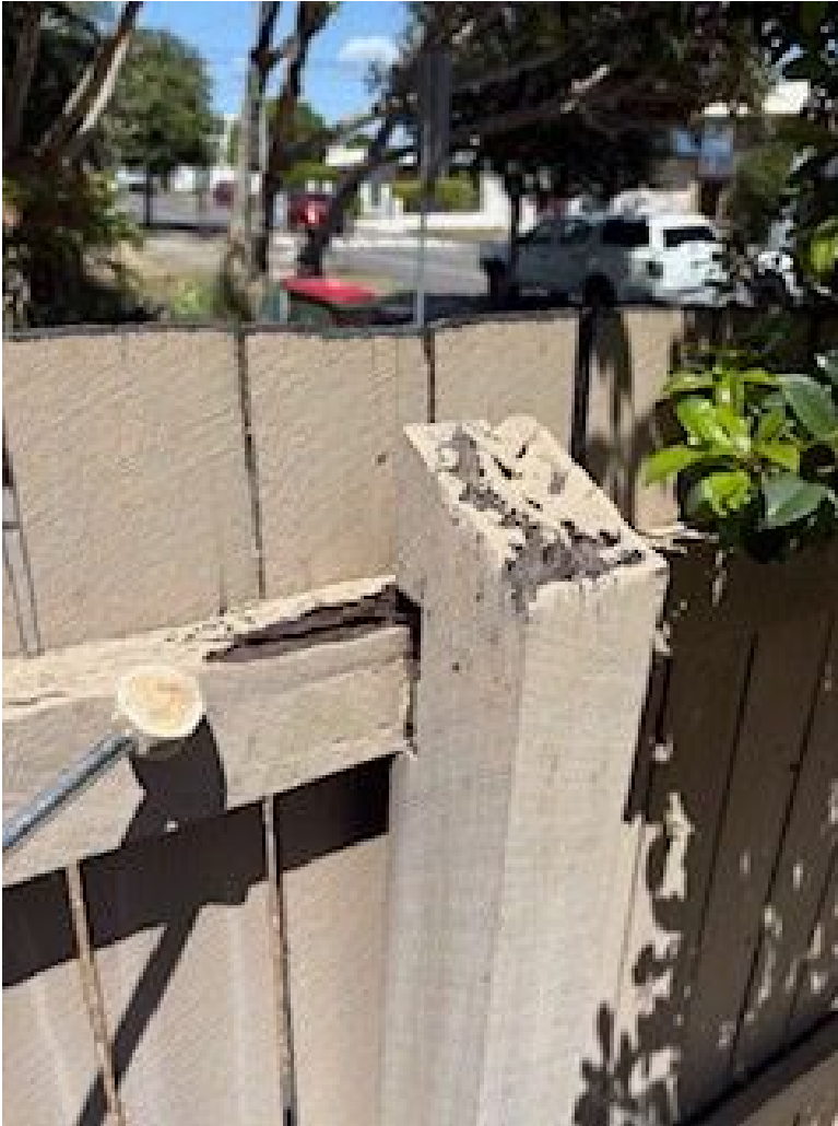
Image comments: Example of fungal decay along the boundary fence.
