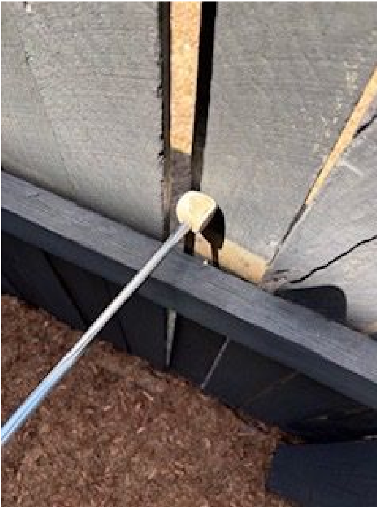
Image comments: Example of a loose piling.
