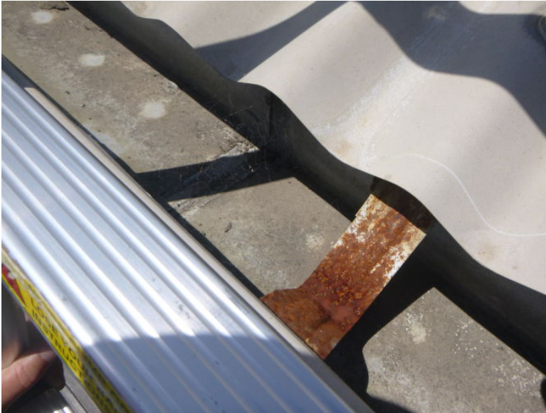
Image comments: Example of surface corrosion of the gutter brackets.
