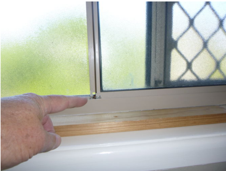
Image comments: Bathroom, sliding sash window, broken joint, bottom left of the frame.
