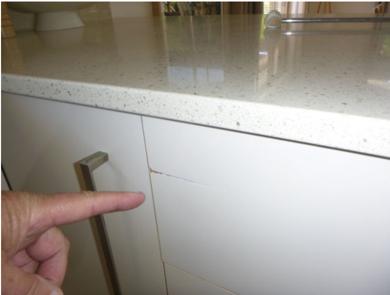
Image comments: Drawer front scratched, adjacent door causing this damage.
