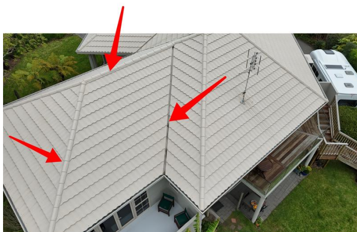
Photo 6 Ridge, hip and valley flashings.
