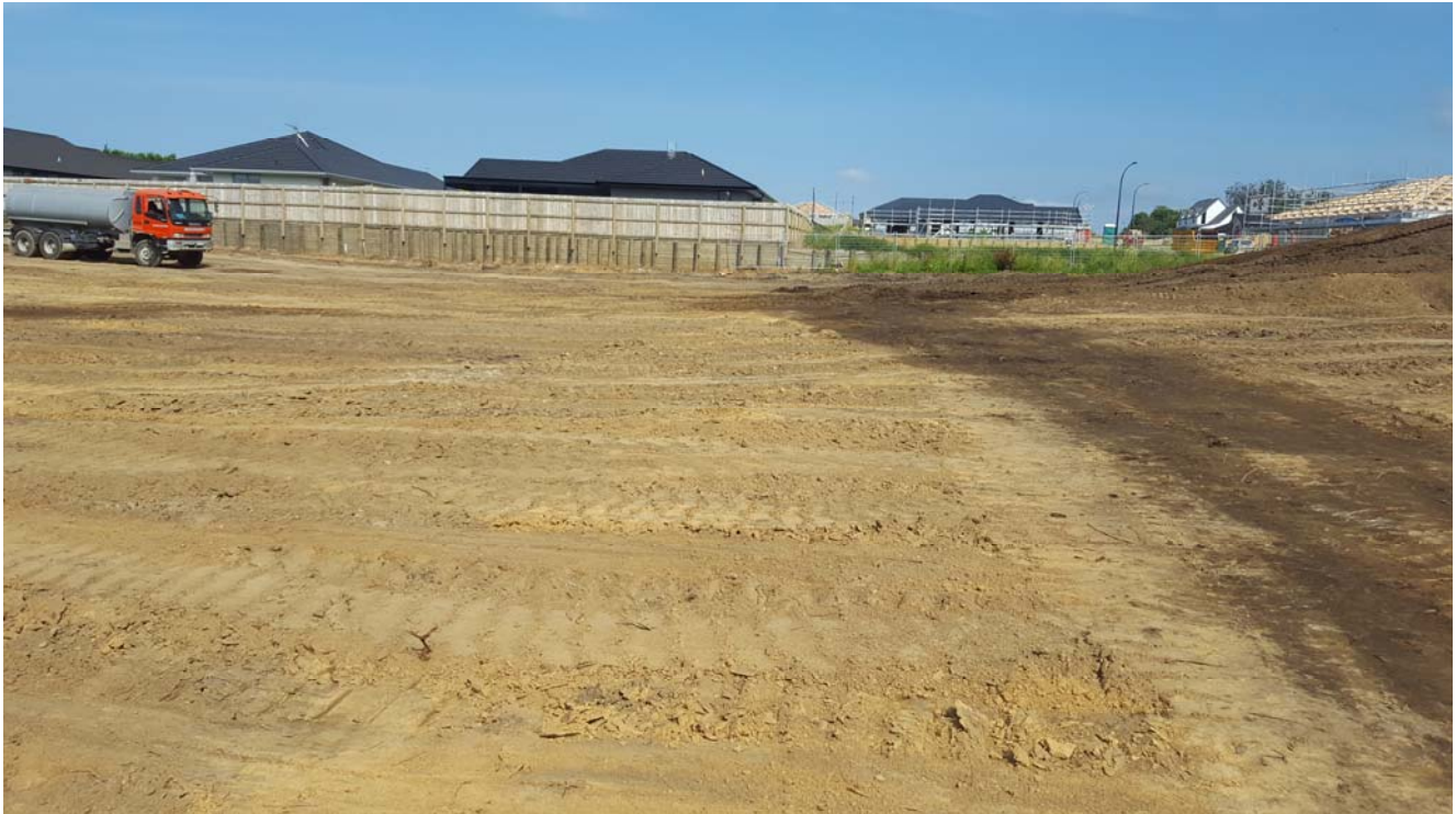
Figure 1: Photo taken facing south east.
