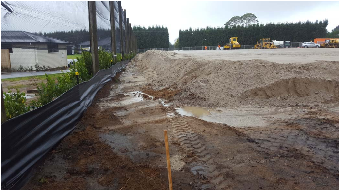
Figure 3: Battered fill behind lots 1 - 6. Photo facing north east.
