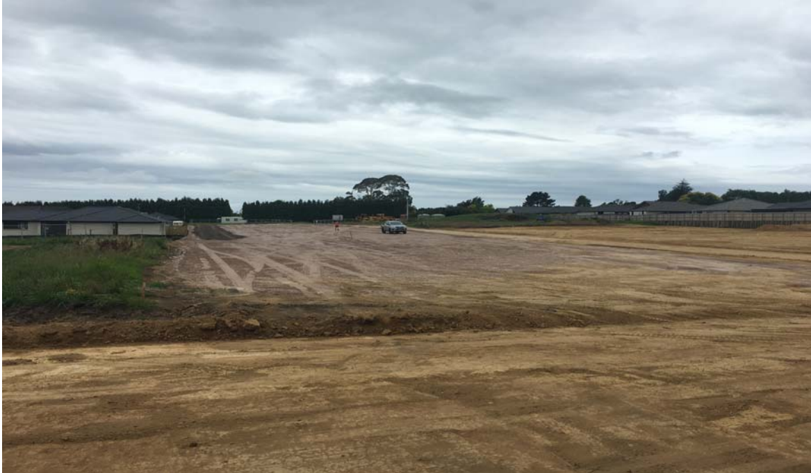
Figure 1: Photo showing extent of fill Photo facing north.
