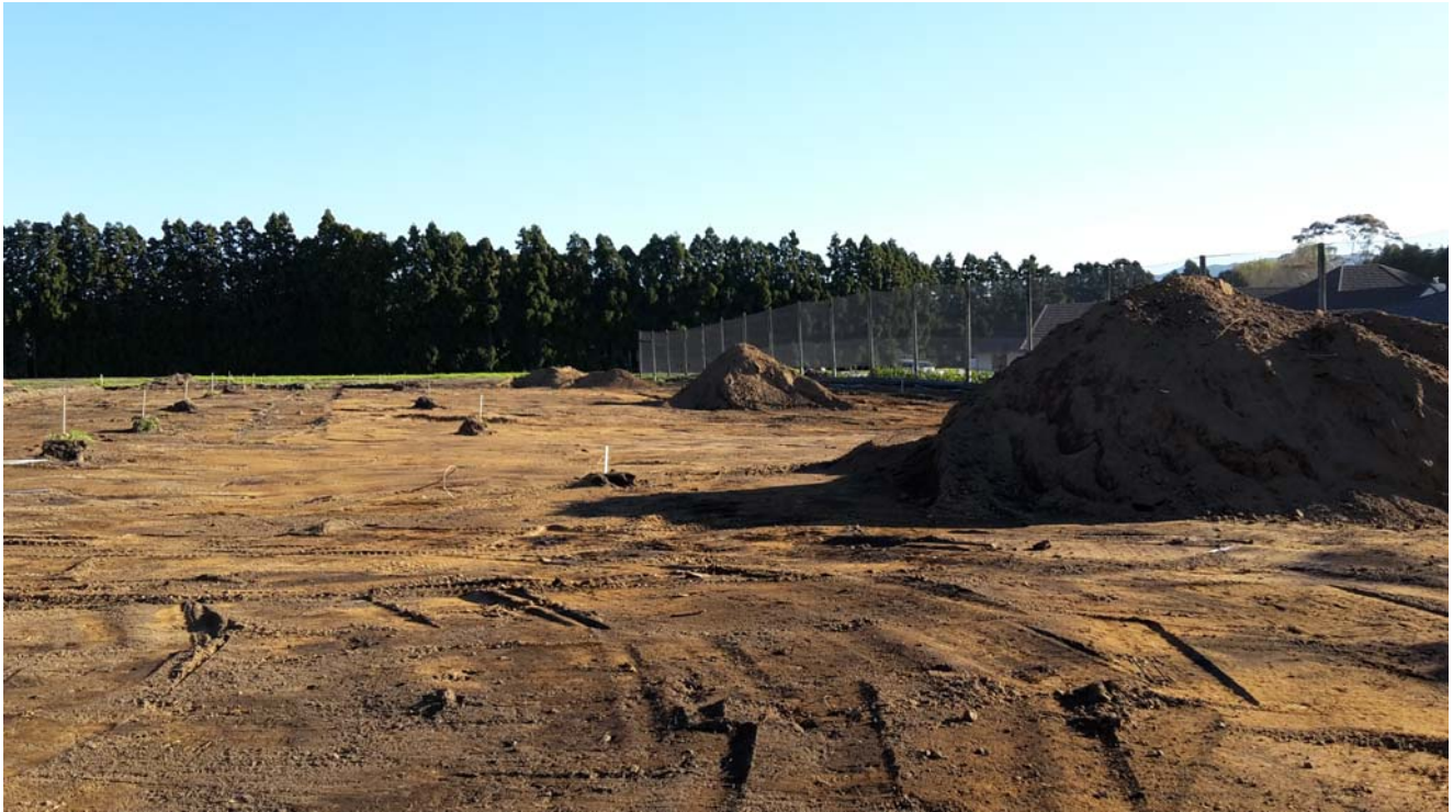
Figure 1: Photo taken facing south west.
