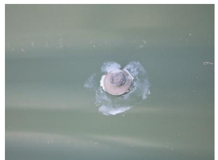
Note these photo examples of the silicone use to some roof fixings
