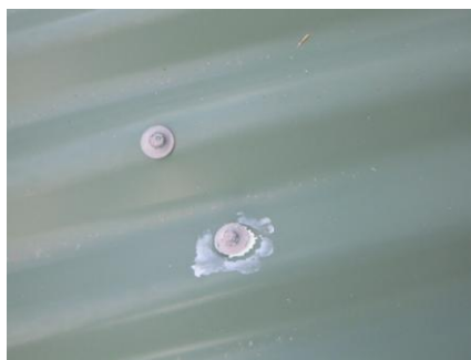
Note these photo examples of the silicone use to some roof fixings
