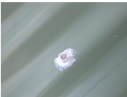
Note these photo examples of the silicone use to some roof fixings
