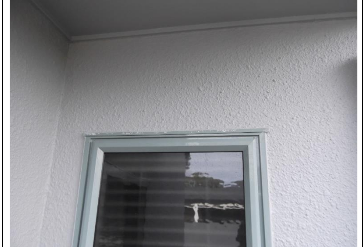
Correct flashings in place. Well maintained cladding
