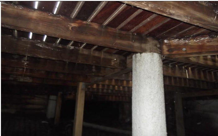
Underside of deck showing sub floor framing
