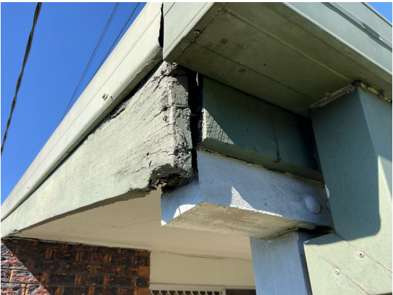
Wood decay (fungal decay) found along the fasciaboards around the home, recommend repairs.
