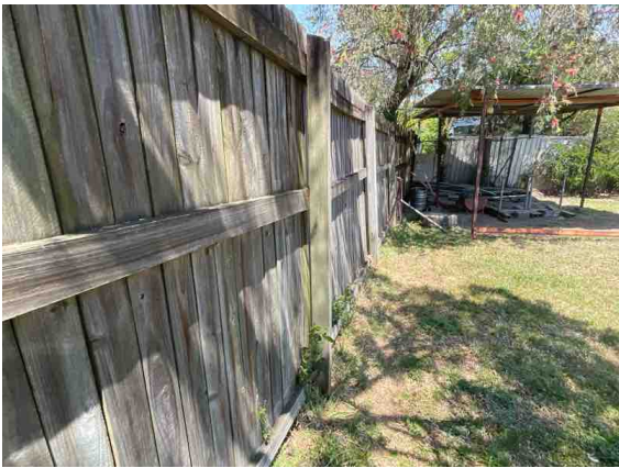
Wood decay (fungal decay) found along the rear fence line, recommend repairs.
