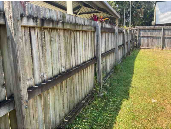
Wood decay (fungal decay) found along the left hand side fence line, recommend repairs.
