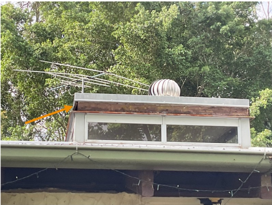
Wood decay (fungal decay) found along the timber fasciboard on the roof, recommend repairs.
