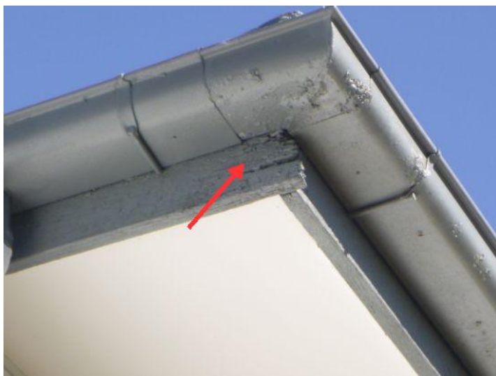
Northwest corner timber fascia
