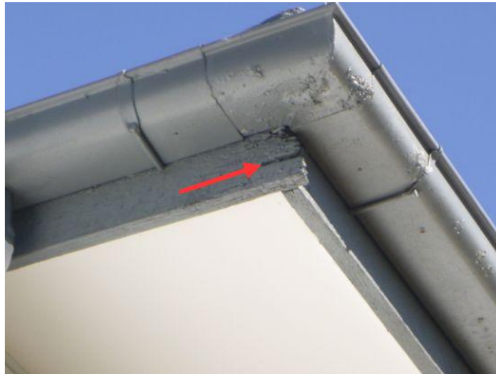
Northwest corner timber fascia
